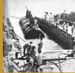
1947 Machinery from Denmark for the Sankarnagar plant arrives at the Tuticorin Port.
