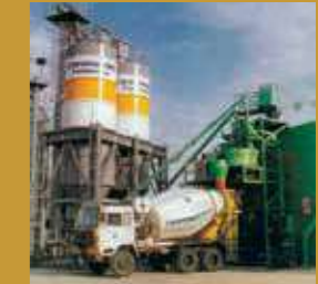
1999 The company's first Ready-Mix Concrete plant in Thirumudivakkam, Chennai.
