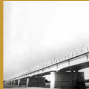
Adur Bridge, Kerala
